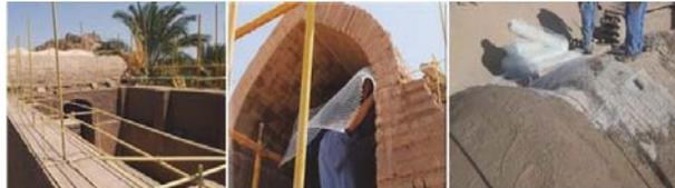
**Figure 4.** Increasing the integrity of roofs and walls by ring beam and stabilizing inner and outer parts of roofs in Sistani House with installing fiberglass mesh (Source: archive of RPBCB, 2008).
