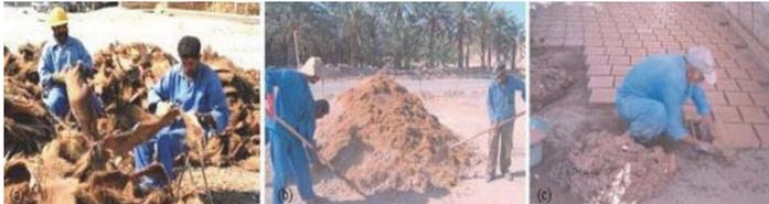
**Figure 2.** Process of the production of reinforced adobes with palm fiber in Bam Citadel workshop
