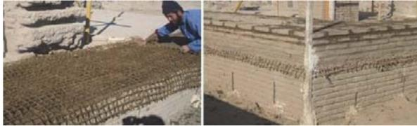
**Figure 7.** The process of Palm mesh insertion between layers of adobe-wall in Payambar Mosque (Source: RPBCH, 2008).
