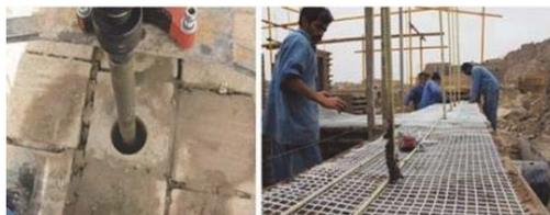
**Figure 3.** (Left) drilling of adobe wall for insertion of fiberglass rods; and (Right) placement of fiberglass mesh on the wall
